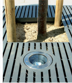
Recess for spotlight
