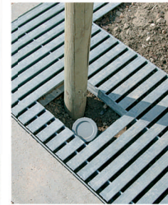
Hatch for stake + drainage
