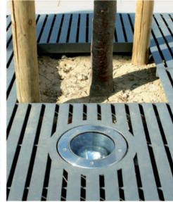
Recess for spotlight
