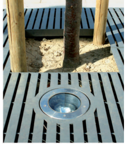
Recess for spotlight
